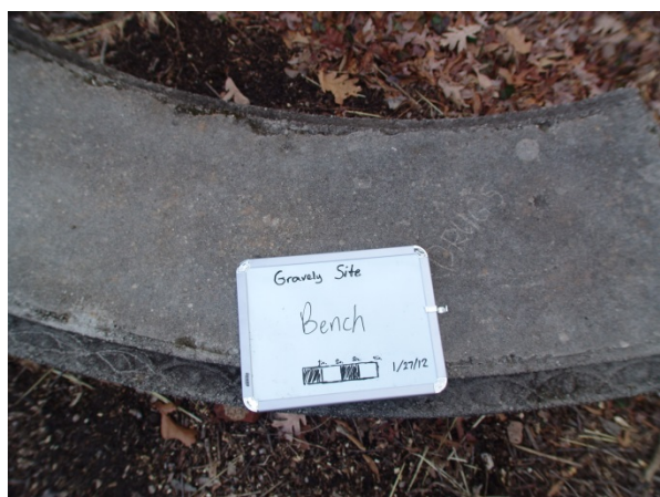
I. Concrete bench
